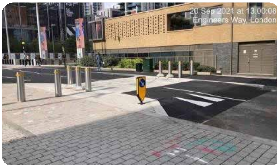
Image 8: Example of one of the HVM Measures on Engineers Way (Source: LBB)
